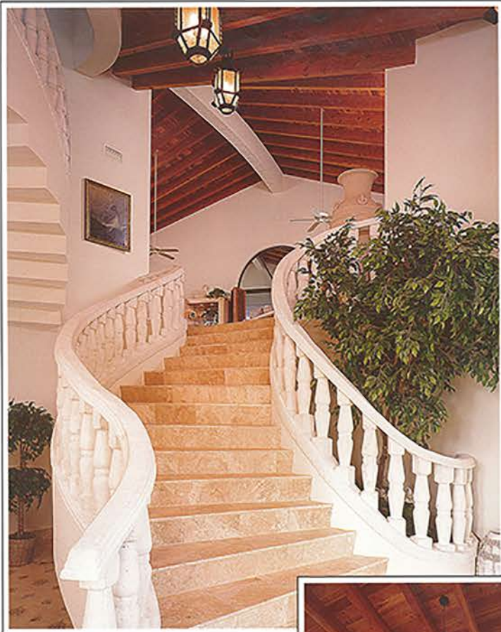
A winding stairway with travertine steps and curving, cast stone railings sets a tone of graceful elegance.
