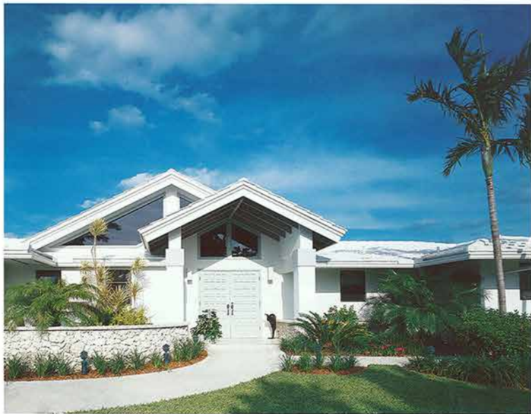
Originally a fishing retreat with a low, flat ceiling, this home was redesigned for volume and to capture views.
